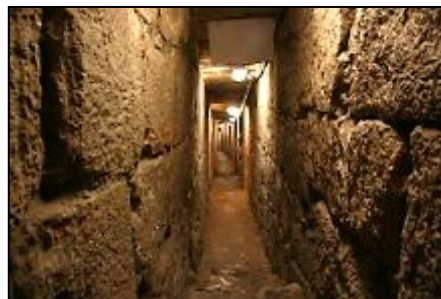
Storm drain that runs under the entire road
